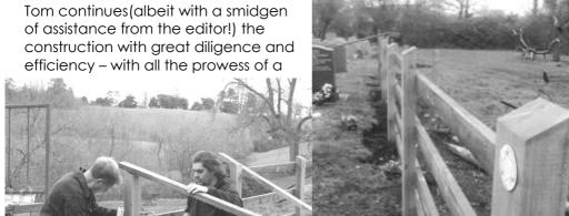
badger and the stamina of a thoroughbred, each post hole is dug by hand to a spade's length depth. Each rail measured and set straight – every angle and gradient checked and assessed. Keep it up chaps, we might see if finished before the end of the magazine... The PCC thank John Hembrow for allowing access and use of his field whilst work was undertaken.
